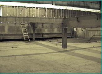
After the existing concrete floor was removed, the structural floor steel was left in place to provide needed support to roof columns during the foam concrete fill making compaction of conventional materials very difficult with equipment. Once the backfill reached the floor steel elevation the floor structural steel members were removed since the foam concrete now provided the lateral support for the roof columns.
