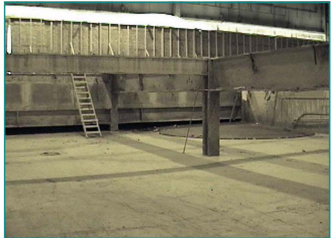
After the existing concrete floor was removed, the structural floor steel was left in place to provide needed support to roof columns during the foam concrete fill making compaction of conventional materials very difficult with equipment. Once the backfill reached the floor steel elevation the floor structural steel members were removed since the foam concrete now provided the lateral support for the roof columns.
